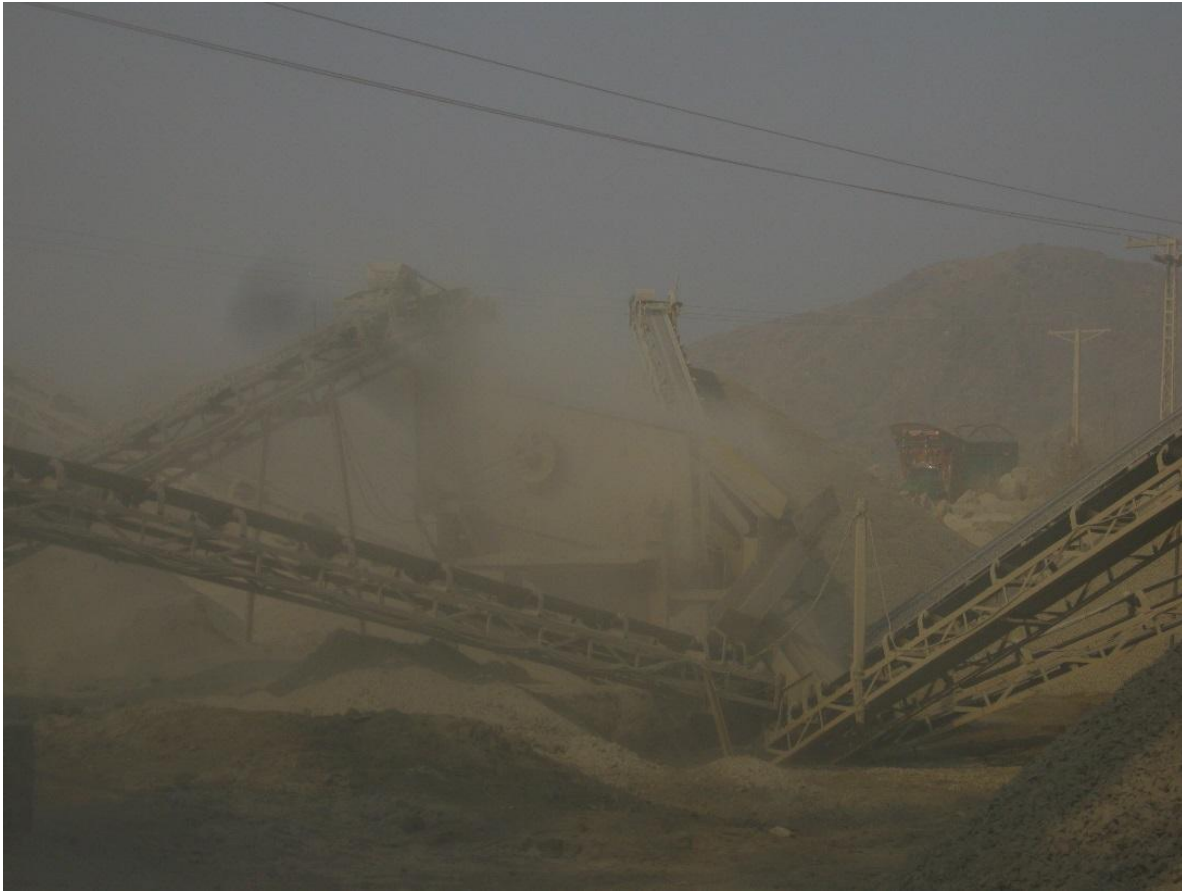
Fig. 3. Crushing units of Sargodha stone crushing industrial area (Pull-111) causing air pollution
